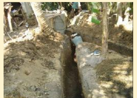
Taking trenches for making radials
